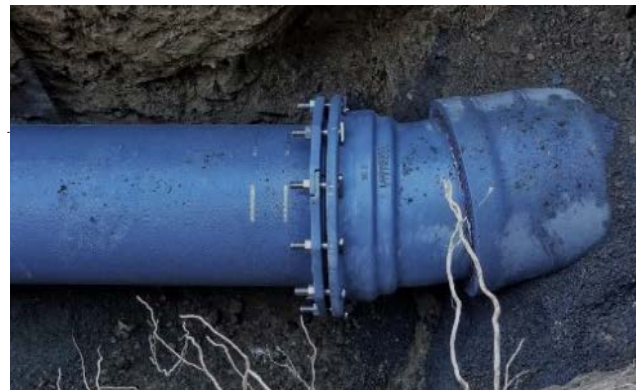
FIG. 6 An example of DN375 x 11 degree bend showing: 1. Type NS Mechanical Bend, Tee Bolts and Gland plate. 2. Type NS mechanical bend socket installed into Type NS Pipe Socket.
