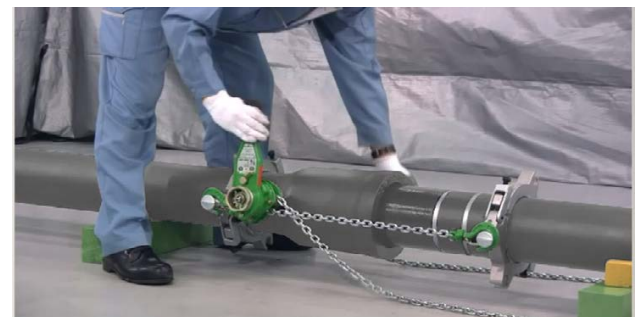
FIG. 7 Type NS pipe joint being made using special tools.
