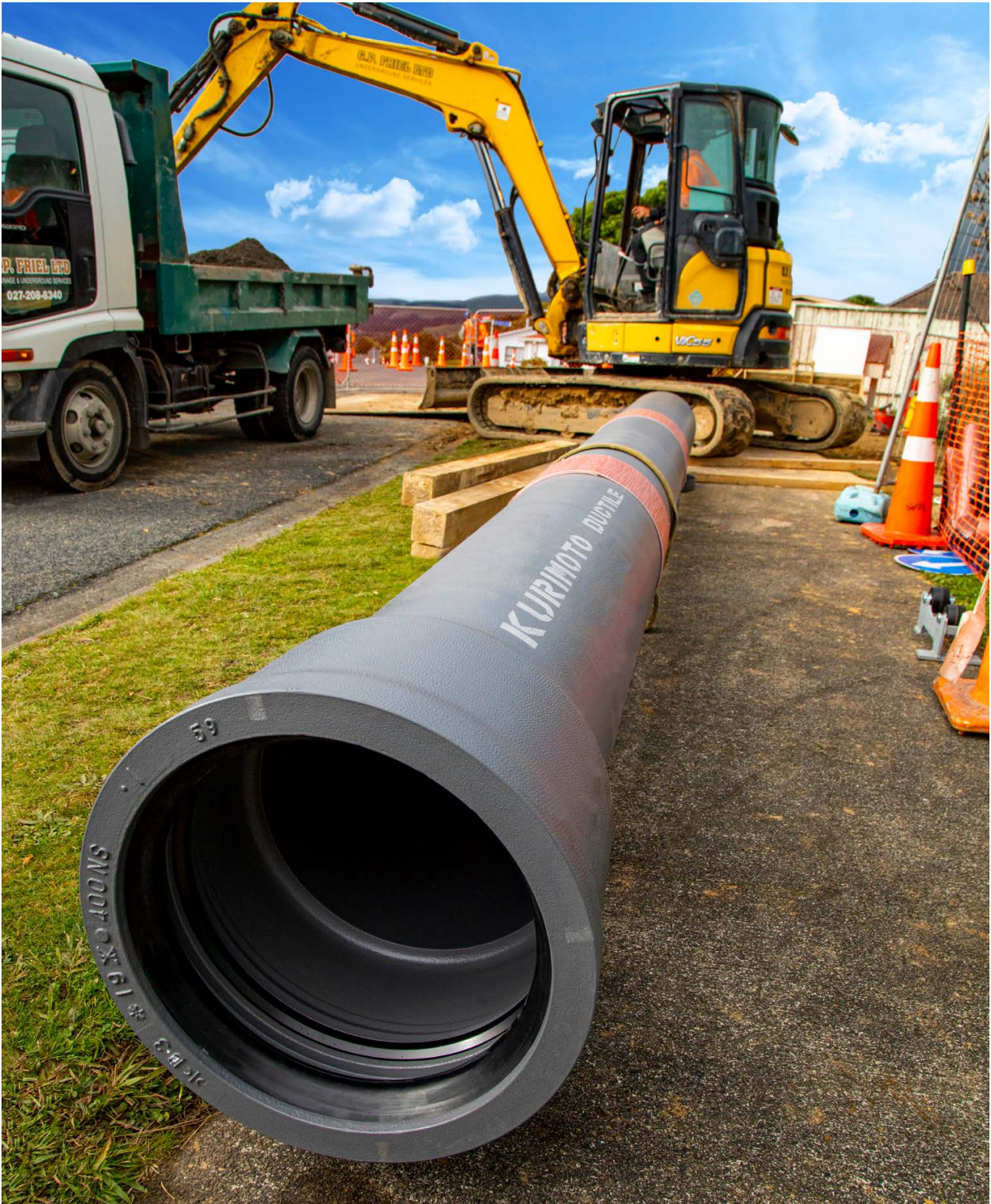
FIG. 14 Kurimoto Ductile Iron Pipe installation in Wellington
