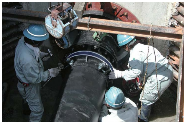
FIG. 12 Work in progress.
