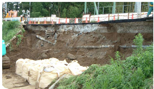
FIG. 4 SRDIP pipe remaining in tact during the 2011 Japan Earthquake
